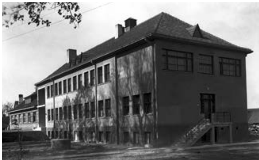
Figure 5. New building of Telšiai hospital, 1940s (Samogitian museum “Alka”)
