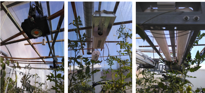
Figure 1. LED COB Helle Top LED 280 luminary, induction lamps and high-pressure sodium vapor lamps Helle Magna (from left to right)
